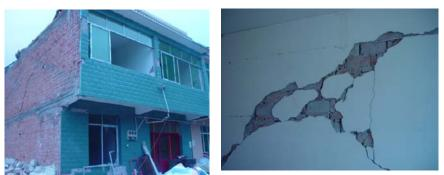
The damaged building shown in Fig.14a) was a self-built two-floor masonry house building, it located at Leigu town, Mianyang county, its geographic coordinate is  $31^{0}47'$  N,  $104^{0}25'$  E. The designed seismic intensity of the buildings in Leigu town is 7 (Ms), the basic designed acceleration of ground motion is 0.10g, it is classed into the first group of design earthquake, and the seismic intensity there is degree X
