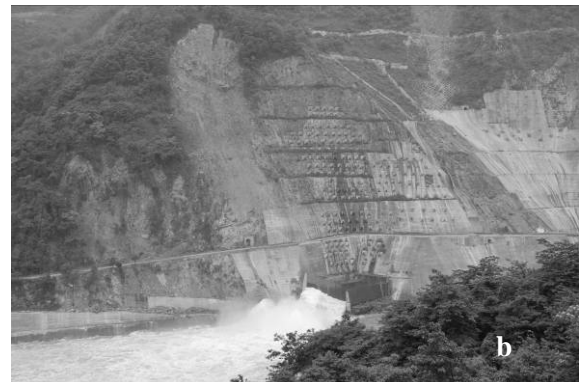
Figure 5: View of large-scale landslides that formed natural dams and lakes along the river course (a) and view of a landslide triggered above the exit of the Zipingpu dam's emergency spillway causing considerable damages (b).
