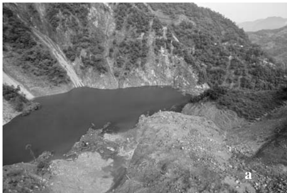
Figure 5: View of large-scale landslides that formed natural dams and lakes along the river course (a) and view of a landslide triggered above the exit of the Zipingpu dam's emergency spillway causing considerable damages (b).
