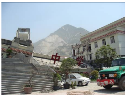
Fig. 1 Collapsed school building in Yingxiu Town (7/11)*
