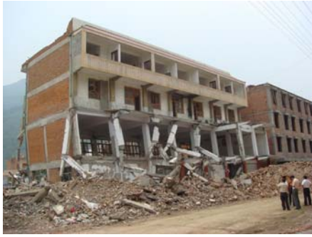
Fig. 3 Two buildings side by side in Pingwu County (7/9)
