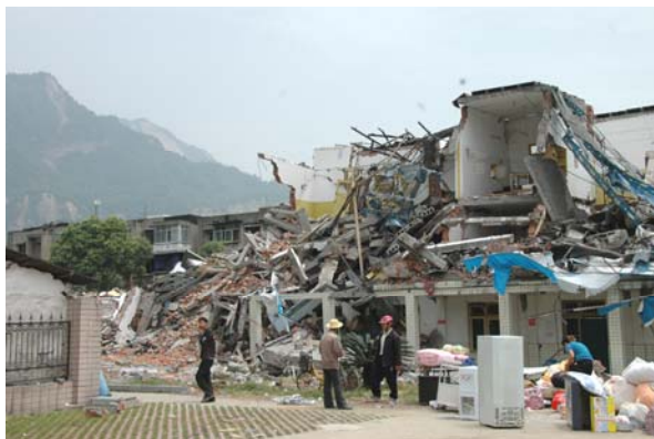
Figure 24 Collapsed Employee Dormitory of the 3 rd People's Hospital at Hanwang township, Mianzhu County after major aftershocks.
