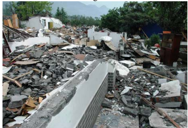
Figure 13 Collapse of traditional houses at Mianzhu.
