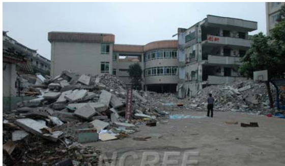
Figure 2 Collapse of elementary school buildings at Dujiangyan.
