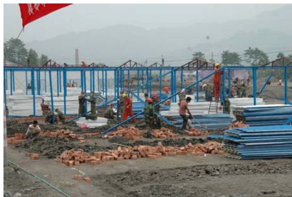
Figure 40 Temporary houses under construction near Pongzhou.
