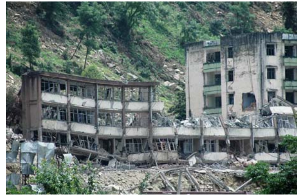
Figure 11 Collapse of residential buildings at Yingxiu.
