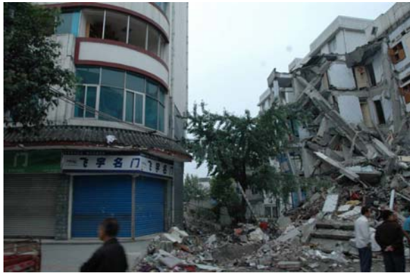
Figure 8 Collapse of commercial-residential buildings at Dujiangyan.
