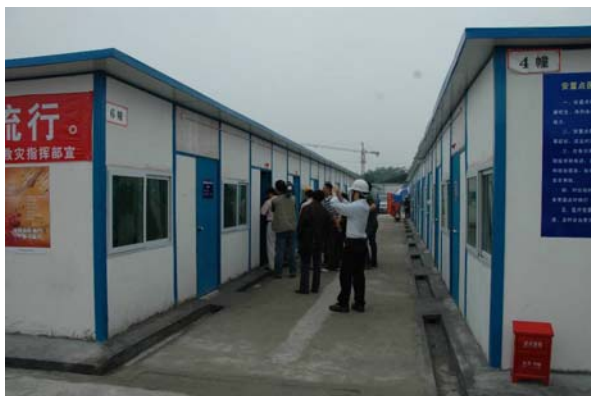
Figure 39 Community of finished temporary houses at Dujiangyan.
