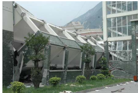
Figure 19 Building collapse due to joint failure.
