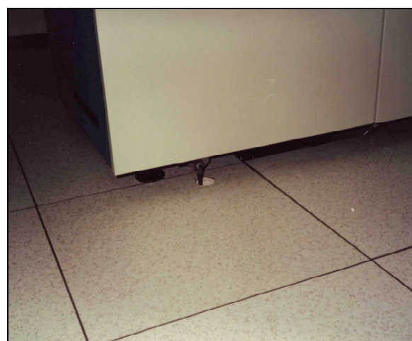
Figure 9 This shows one corner of the cabinet with a cable anchoring method. A turnbuckle below the raised floor allows the cable to be tightened to reduce movement.
