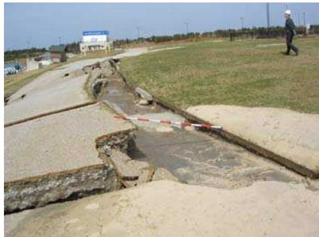
Photo 2 Flow failure of the ground at Uminonakamichi Seaside Park
