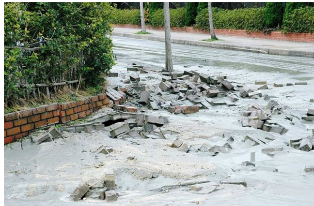
Photo 1 Location of sand boils in the residential area of Atagohama(provided by Ms. kayoko Hoshiko)
