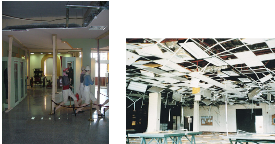
Figure 1 Removing suspended ceiling components for pre-risk analyse of restoration project , fixtures by pillars to protect artifacts at Istanbul Fire Brigade Museum. (left) and Damage to suspended ceiling and recessed ceiling lights, Philippines, Earthquake Engineering Research Institute (right)
