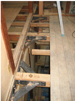
Photo 5. Repairing the cut beams.
