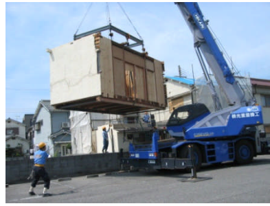
Photo 4. Lifting and transporting.
