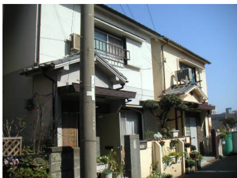
Photo. 1 Exterior view of tested house.
