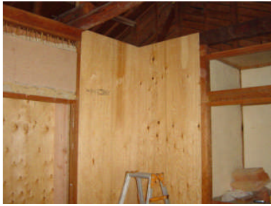
Photo 3. Reinforcement for transporting.
