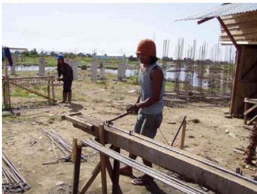
Figure5 Bending works on site with simple tools Fabrication of rebar is also conducted on ground
