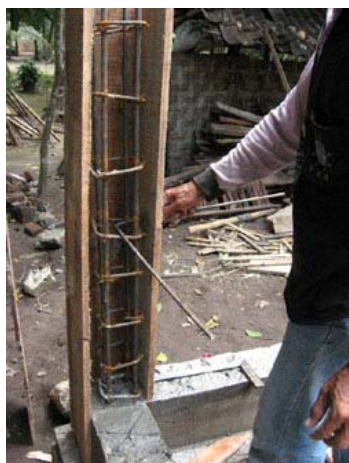
Figure17 Anchorage of walls to column
