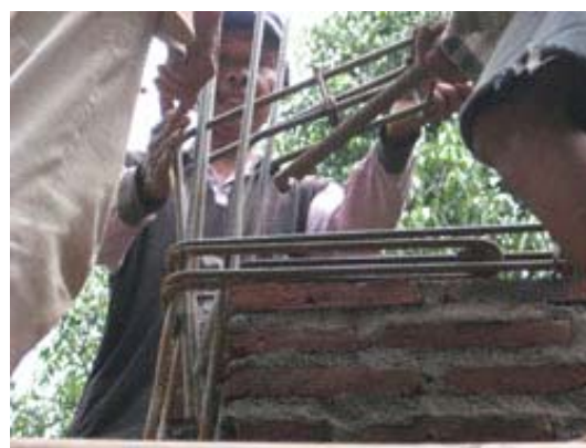
Figure16 Connection of RC members Horizontal rebar is not connected at the corner, but using continuous rebar
