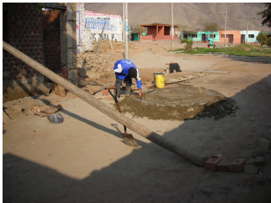
Figure7 Concrete mixing on ground on site Mixing is carried out without sheets or others tools
