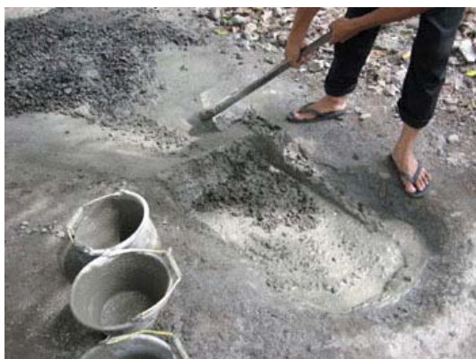
Figure13 Concrete mixing on ground on site Mixing is carried out without sheets or other tools
