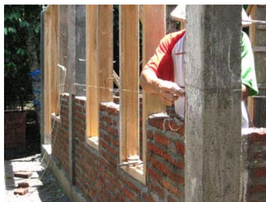
Figure18 Laying work of bricks with taut line
