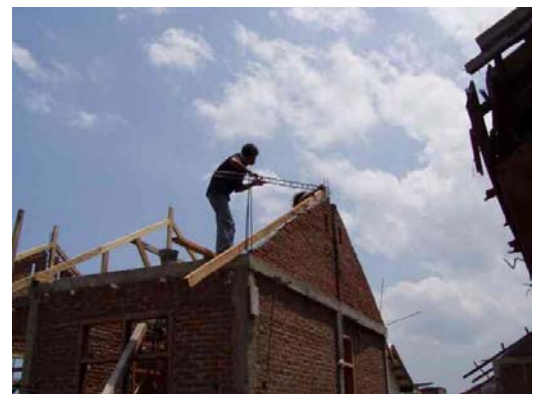
Figure6 Placing rebar of a roof beam fabricated on ground
