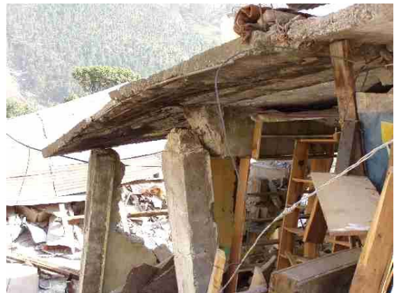
Figure2 Failures often occurred in connections of structural members
