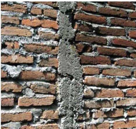
Figure21 Poor concrete placing work with a lot of honey comb and void
