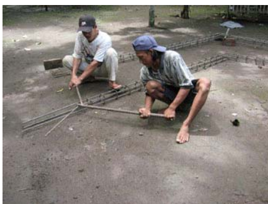
Figure15 Bending works of rebar on ground with simple tools without machines
