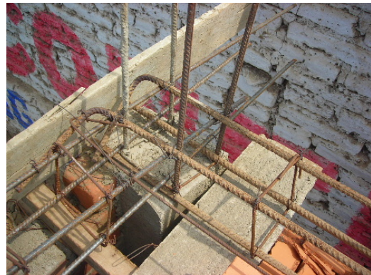
Figure10 Corner of beams and column Length of lapped splices is limited to the dimension of RC members' section size because of fabrication method
