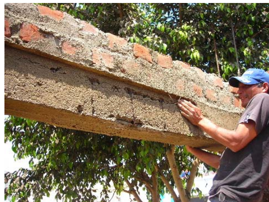
Figure12 Honey comb in beam Some of rebar is exposed to air
