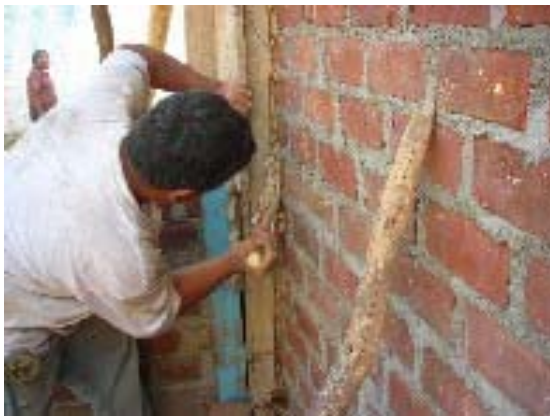
Figure11 Form works Packing of small piece of cement bags is usually observed
