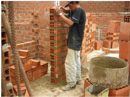
Figure9 Laying work of bricks with plumb bob Taut line is usually used
