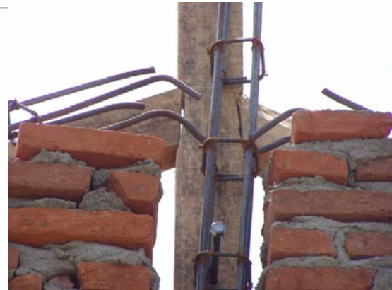
Figure4 Construction practice on site Insufficient connection of longitudinal rebar
