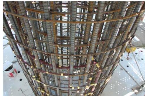
Photo 2 Reinforcements in Three Layers
