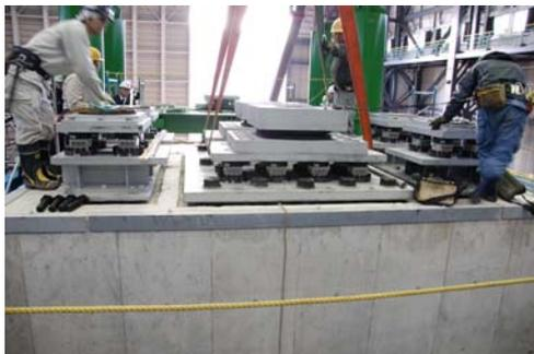
Photo 4 Fixed bearing and 2 Side Sliders
