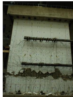
Figure 9: PW3 at End of Test (1.25% Drift)
