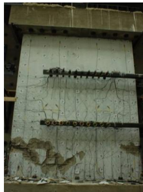
Figure 8: PW2 at End of Test (1.5% Drift)
