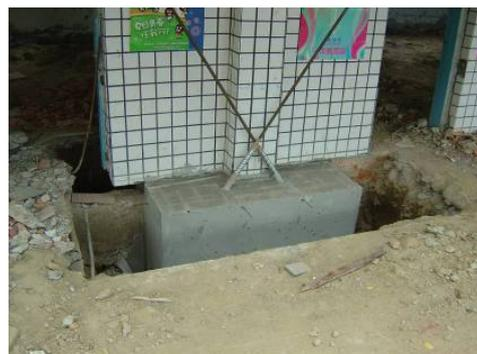
Figure 8 Anchorage block of foundation
