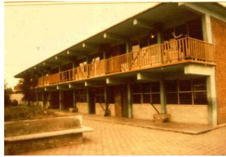
Figure 2 School building retrofitted with PT tendons along the longitudinal direction in Mexico.
