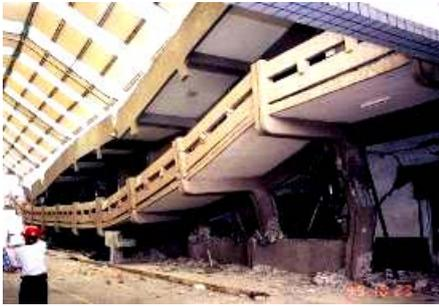
Figure 1 School building was damaged along the longitudinal direction in the 1999 Chi-Chi Earthquake in Taiwan.
