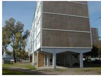
*Figure 1 Photos of soft-storey buildings in Australia*
