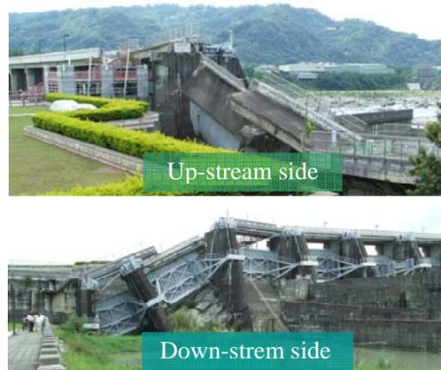
Figure 1 The Shih-Kang Dam damaged by the vertical relative displacement during the Taiwan Chi-chi Earthquake in 1999
