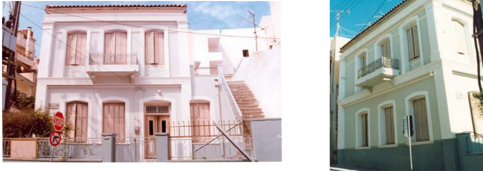
Figure 3 Views of the two stories Building in Kazantzaki Street in Sitia
