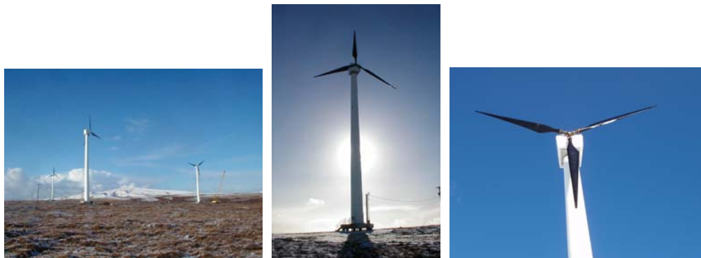
Figure 1 Operational wind towers
