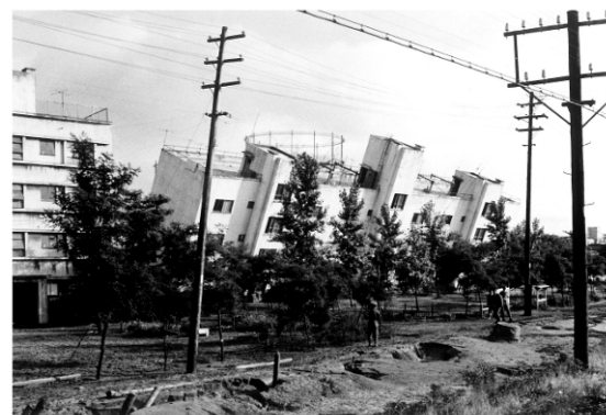
Figure 14 Tilting of Kawagishi-Cho Apartment buildings
