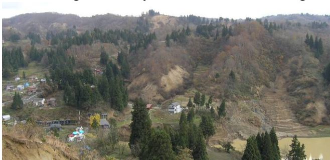
Figure 3 Location of houses and slope failures (2004 Niigata-Chuetsu earthquake)
