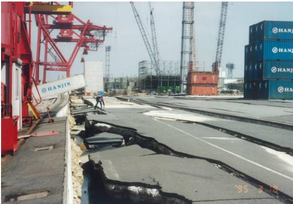
Figure 21 Liquefaction in Kobe Port Island
