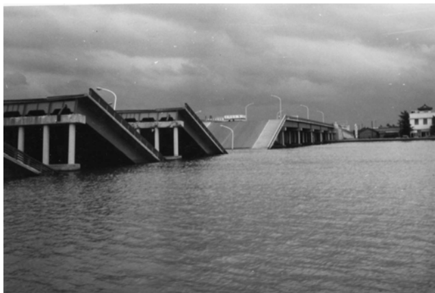
Figure 15 Liquefaction-induced collapse of Showa Bridge
