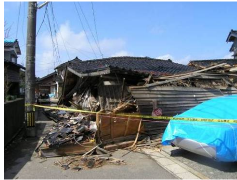
Figure 2 Damaged wooden house (2007 Noto earthquake)
