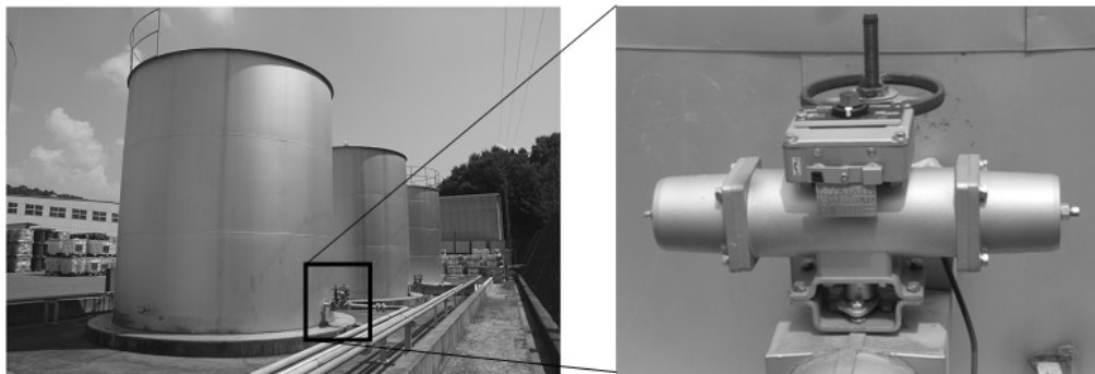
Photo 2 Example of shutdown system by a valve attached to a tank of toxic materials.
