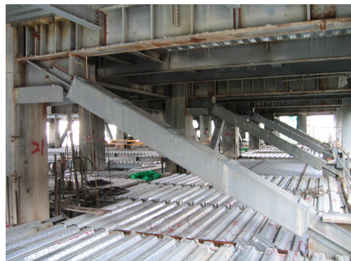
Fig. 10 Installation of the BRBs in the construction site
