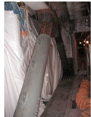
Photo 1. Seismic control braces
