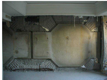
Fig. 10 Double-X shape buckling restrained brace
