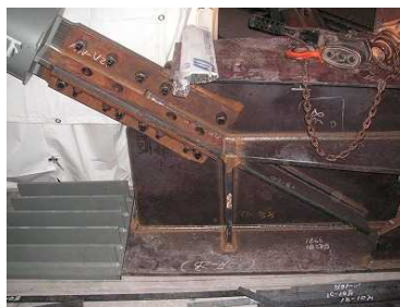
Photo 2. Seismic control brace joint
