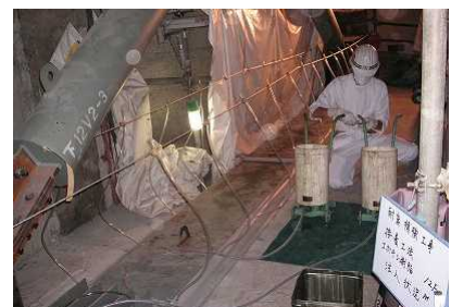
Photo 3. Epoxy resin being injected
