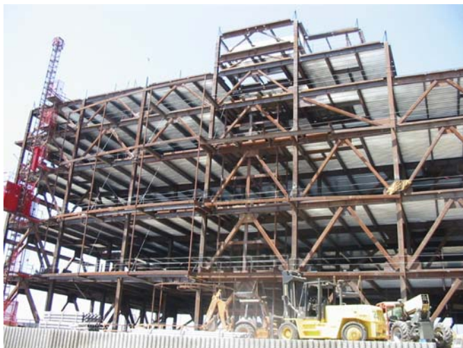
Figure 7 LARTMC bracing scheme (SCBF)
