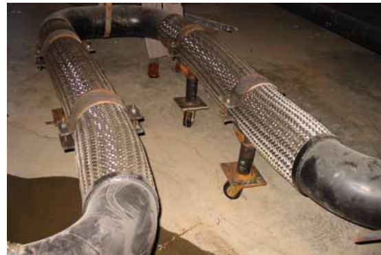
Figure 10 Flex utility joint accommodating a displacement of 24in
