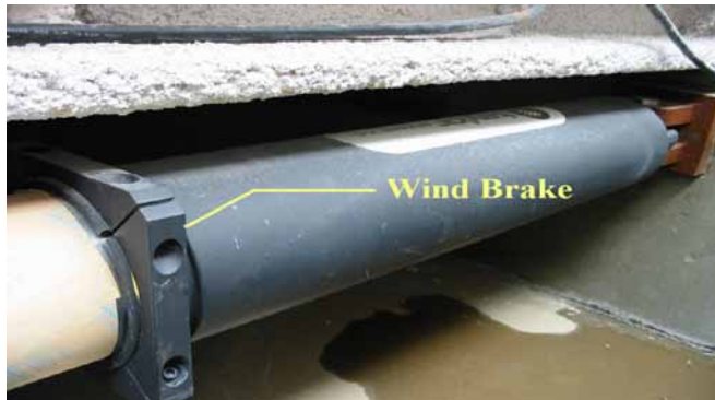
Figure 9 Installed 320kip VFD with wind brakes
