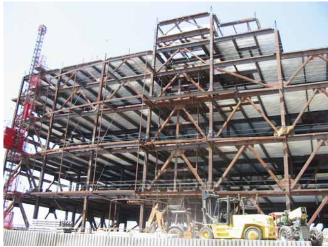
Figure 6 LARTMC bracing scheme (SCBF)
