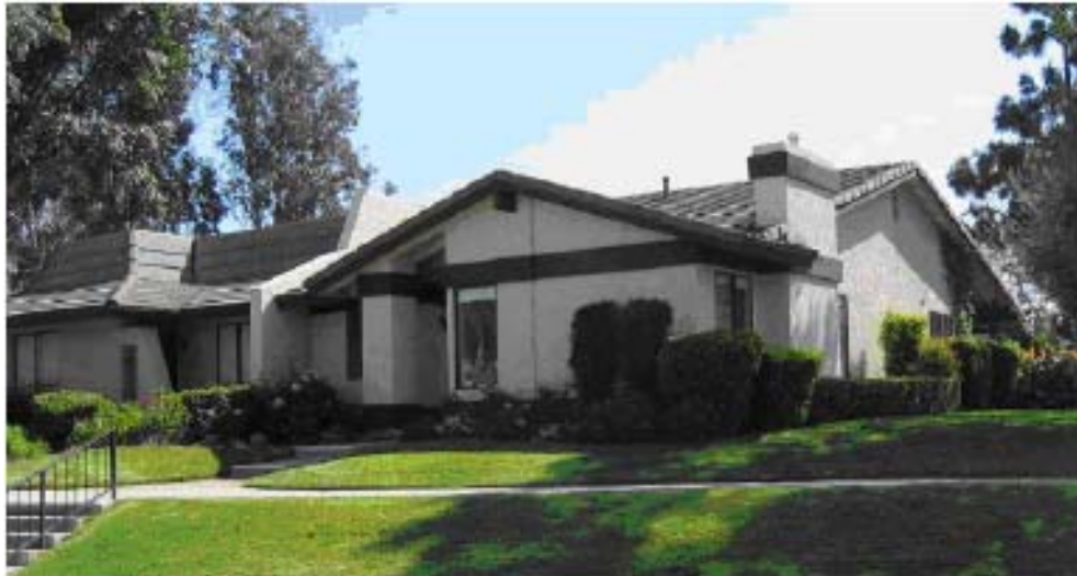
Figure 1. Subject building: typical 1970s construction in southern California
