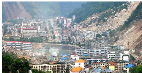
Fig. 1 Beichuan Town was nearly buried by landslips
