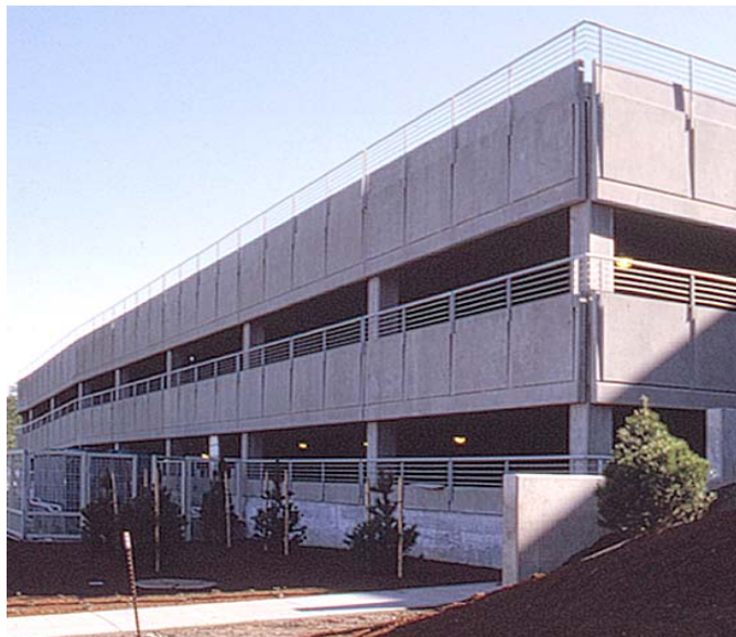
Figure 2. Parking garage concept. Open structural systems allow water to pass through with minimal resistance, and interior ramps allow for easy ingress and vertical circulation.
