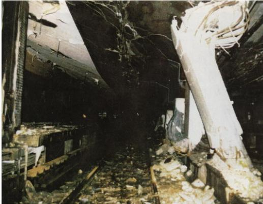
(a) The real seismic damage of the Daikai station
