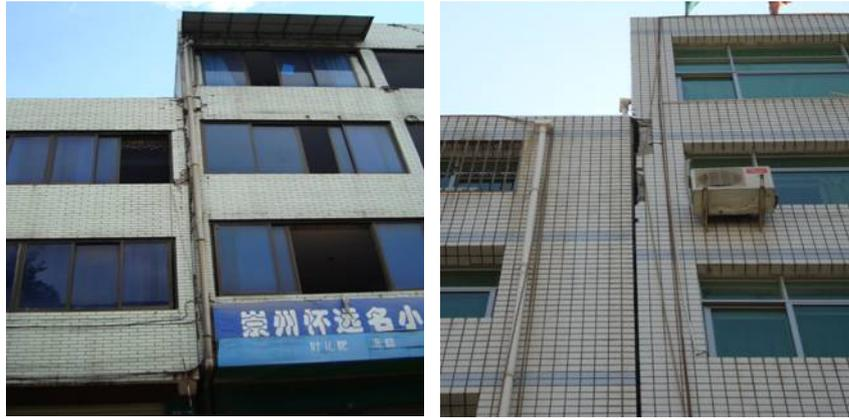
Figure 1 Damages caused by pounding during the M8.0 Wenchuan earthquake on May 12, 2008
