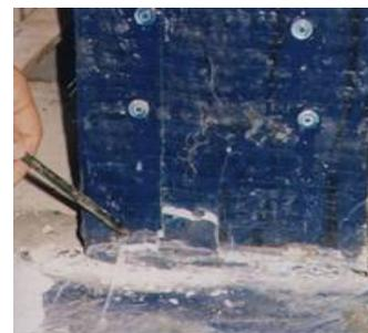
**Fracture of CFRP at the joint between the pier and the foundation**
