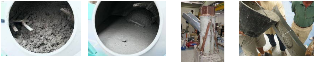
Figure 5. (a) SCC production (b) formwork (c) SCC jet process.
