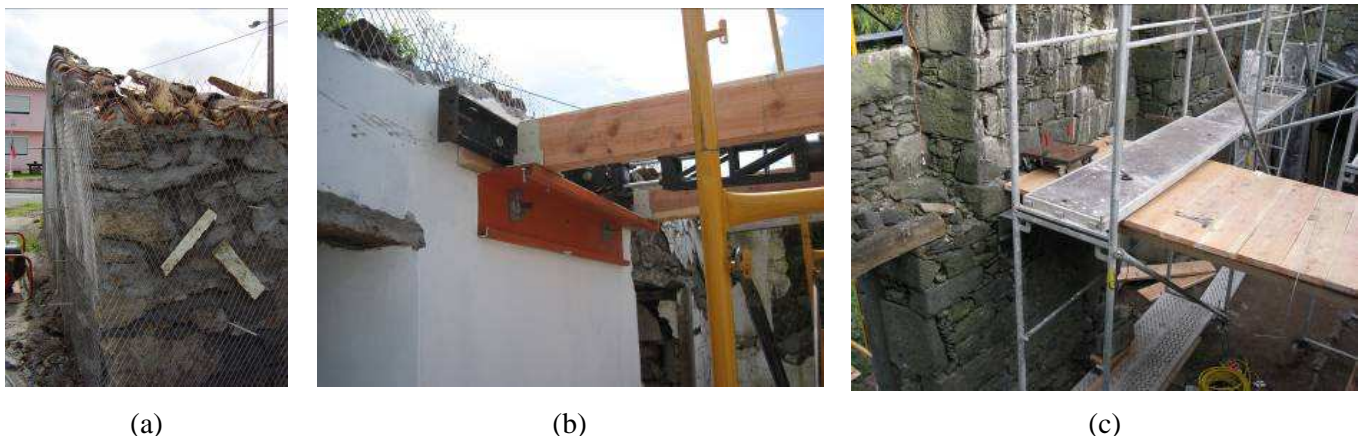
Figure 7 Strengthening schemes: (a) steel reinforced mortar cover in masonry walls; (b) wood beams supported and fixed to opposite walls; (c) wood boards nailed to floor beams to include pavement contribution
