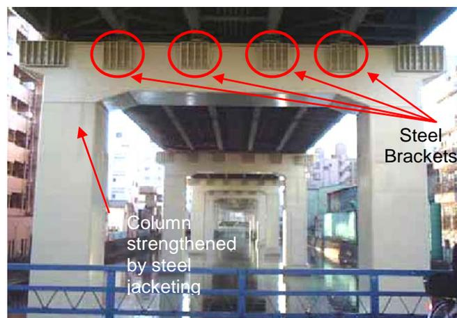
Figure 1 A typical RC frame of a highway bridge in Japan.
