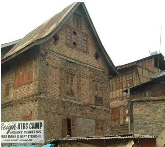
Fig 3. The Kashmir house using Masonry and Timber construction
