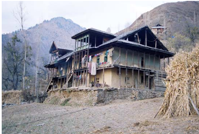
Fig 5. The Kashmir house with its distinct plinth, body and roof.
