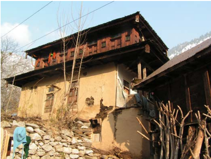
Fig 10. The upper levels of the house are constructed of lighter material.
