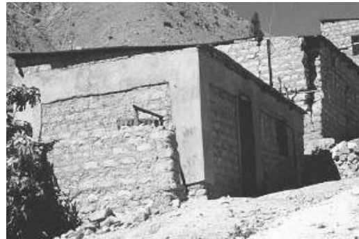
Reinforced house (Arequipa earthquake 2001)
