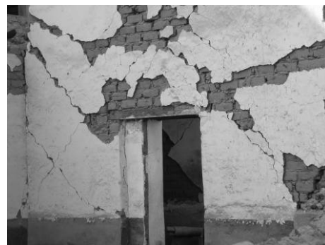
Diagonal cracks
