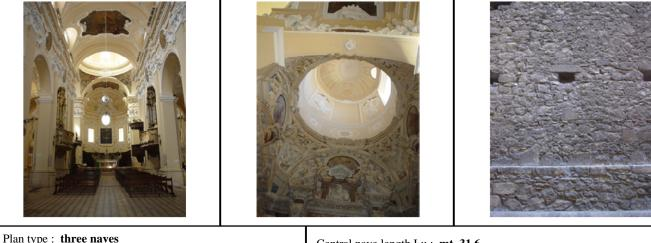
Central nave length Lu : mt. 31,6 Central nave width La: mt. 7,4 Area covered: mq.650 Vulnerability:.0,52 Activation mechanisms:M1- M2- M9- M16- M25- M27- M28
