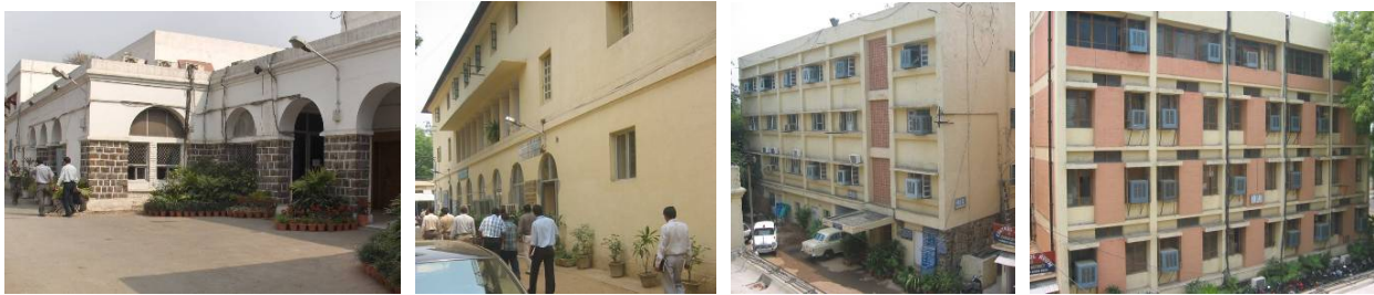
Figure 4. Blocks A, B, C and D (left to right) at the Divisional Commissioner's Office Complex.
