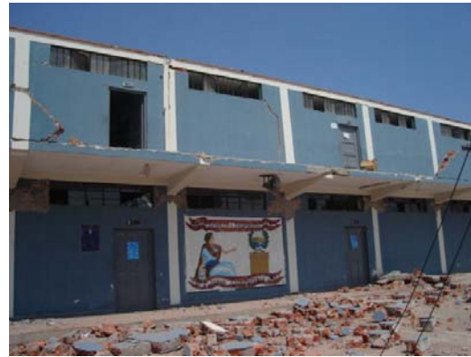
Figure 11. Antonio Skrabonja Social Security Hospital. School building, non structural and structural damage. 1977 design standard. Pisco
