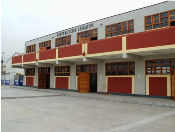
Figure 9. Post earthquake condition of school building designed using 1997 Standard.
