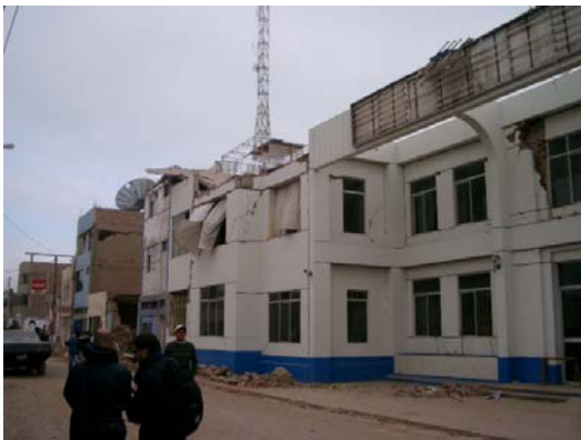
Figure 11. Antonio Skrabonja Social Security Hospital. School building, non structural and structural damage. 1977 design standard. Pisco
