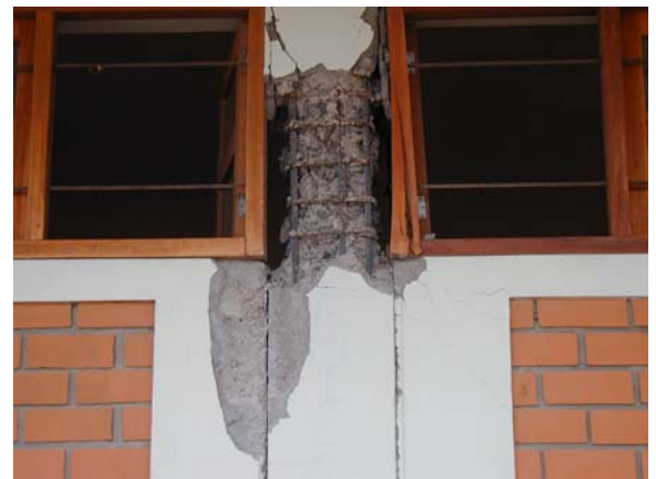
Figure 8. Damage to building designed using 1977 Standard.
