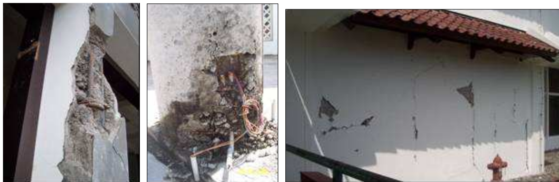
Figure 2. Some structural damages in the UMY campus buildings close to liquefaction locations
