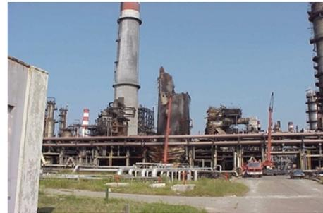
Figure 2 Heater Stacks after Earthquake
