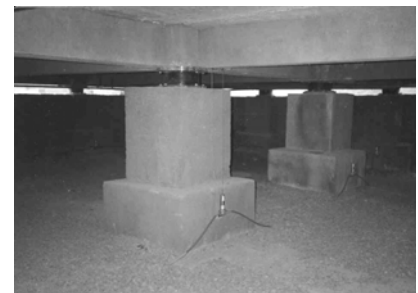
Figure 2 Fragment of base isolation system of four-story newly constructed apartment building in Spitak
