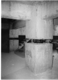
Figure 3 Fragment of base isolation system of four-story newly constructed apartment building in Gyumri
