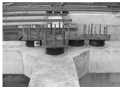
Figure 9 Example of installation of six rubber bearings under one of the columns of the 17-story base isolated building
