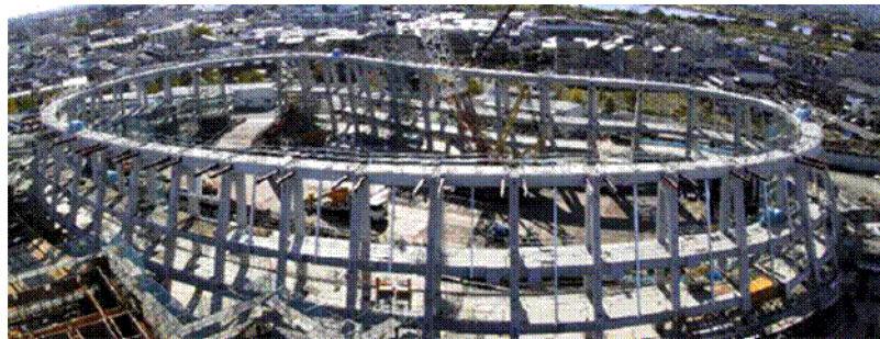
Figure 11: Supporting structure (pre-cast pre-stressed concrete)
