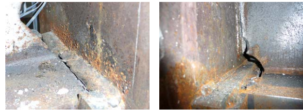
(a) 3F Field weld (b) 3F Shop weld
