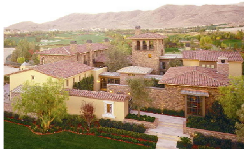
Figure 3 The light wood structure building after finished
