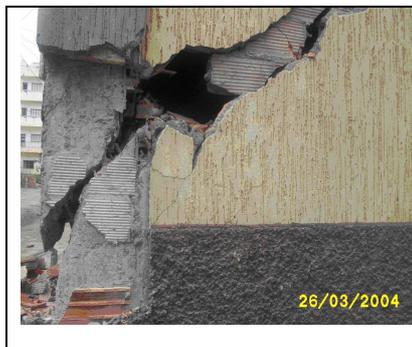
Fig 19 failure of angular column
