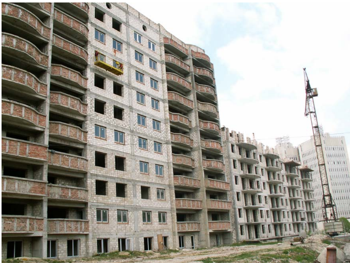
Figure 4. Frame building with filling from sawn lime-stone blocks.
