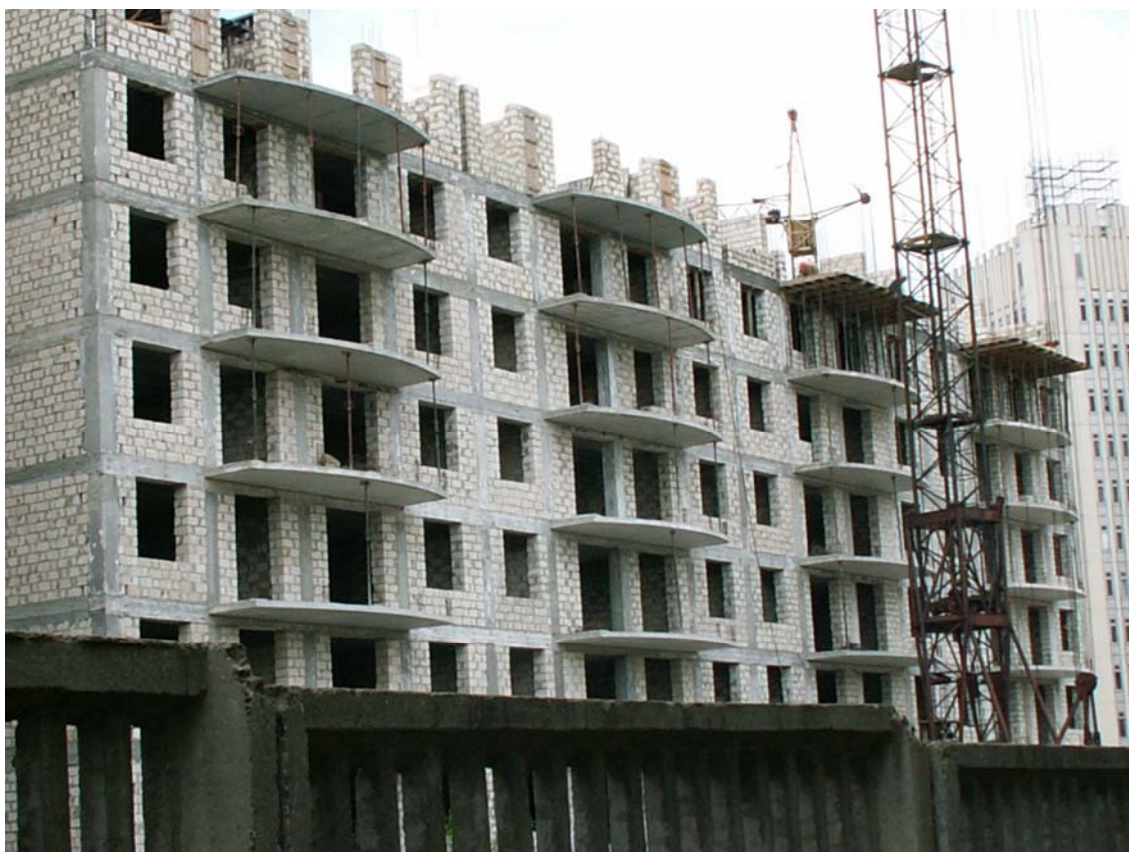
Figure 5. Frame building with filling from sawn lime-stone blocks.
