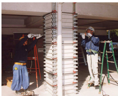
Figure 1.1 Seismic retrofit with stressed external hoops
