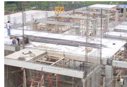
b. Installation of PC-elements
