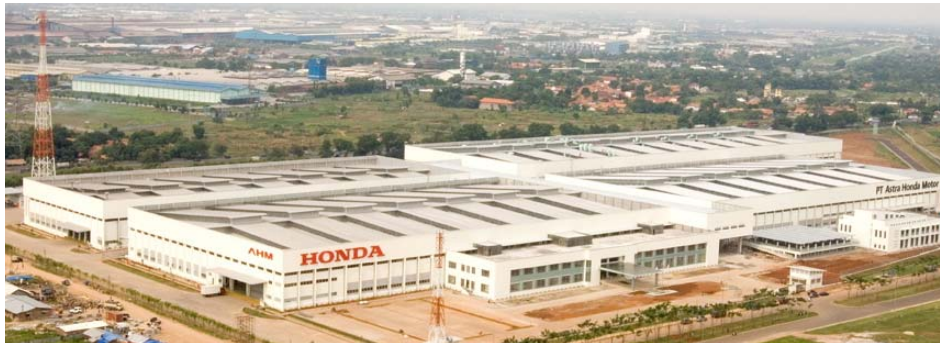
a. Aerial View
