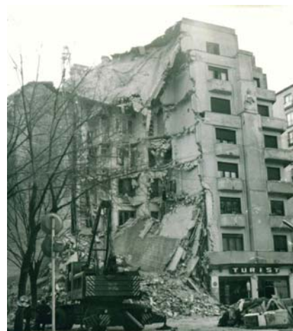
Photo. 1 Severely Damaged Building in 1977 Vrancea Romania Earthquake [JICA Report]
