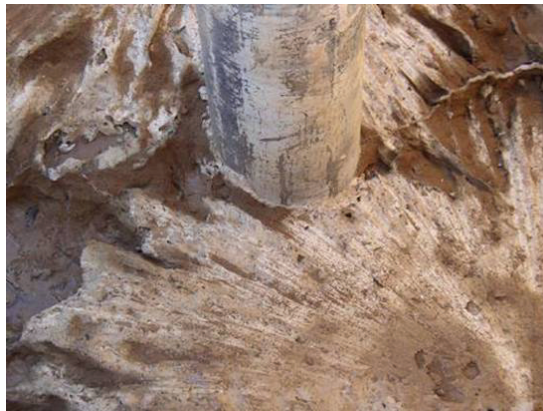
Photo 2 Situation of excavated reinforcement body (pile surrounding status).
