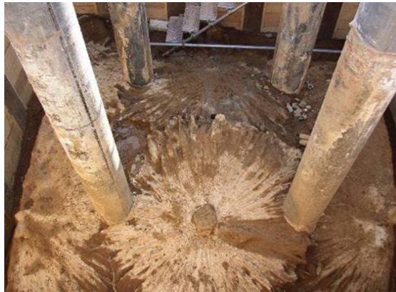
Photo 1 Situation of excavated reinforcement body
