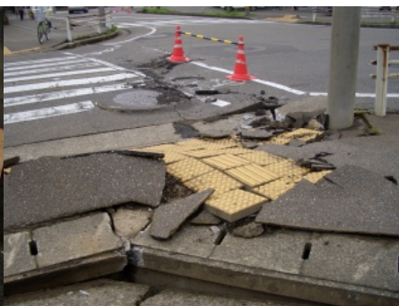
Photograph 10 Damage of asphalt road surface (Kashiwazaki)
