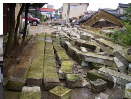
Photograph 6 Collapsed stone masonry walls. The street completely blocked by with both side walls. (Kashiwazaki)
