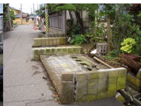
Photograph 8 Concrete block masonry wall with reinforced steel bar and counterfort falling (Kashiwazaki)
