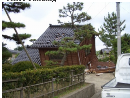
Photograph 16 Collapsed two story warehouse (Kariwa)
