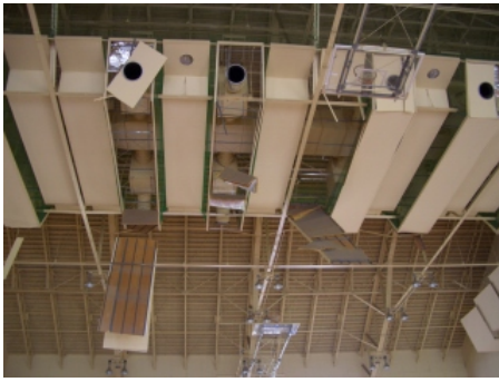
Photograph 22 Damage of ceiling panel of gymnasium in Nishiyama Junior high school(Nishiyama)
