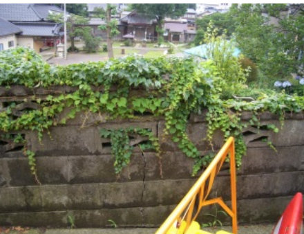
Photograph 32 Crack of concrete block wall (Kakizaki, Joestu)
