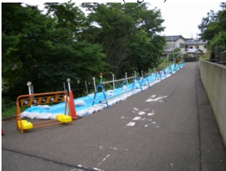
Photograph 31 Blue sheet was covered on the road by surface cracked(Kakizaki, Joestu)
