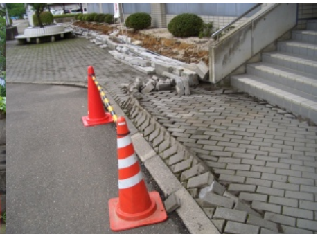
Photograph 33 Damage of Inter Rocking Block(Yoshikawa, Joestu)
