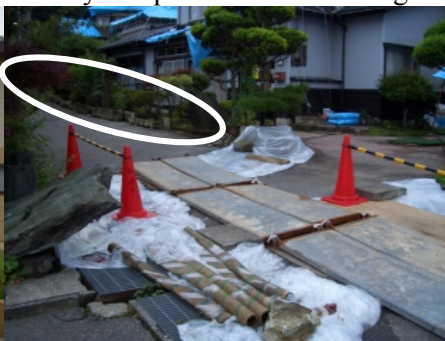
Photograph 20 Concrete block wall falling and road surface gap (Nishiyama)
