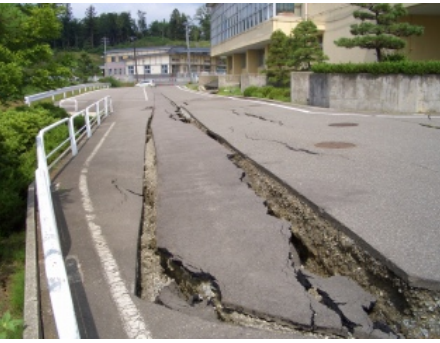
Photograph 23 Gap of asphalt surface front of Nishiyama Junior high school. (Nishiyama)
