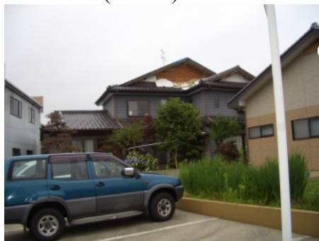
Photograph 19 Cracked gable surface of house (Nishiyama)
