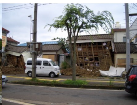
Photograph 8 Heavy damaged warehouse with mud wall. (Kashiwazaki)
