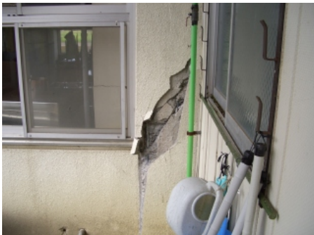
Photograph 28 Shear crack of column of Shimo-Oguni elementary school (Oguni)
