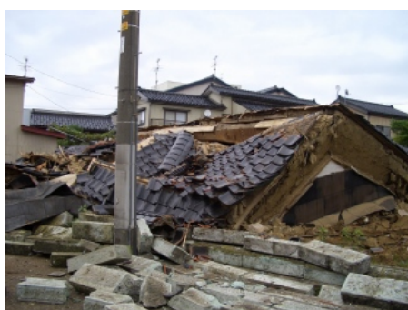
Photograph 7 Collapsed house and stone masonry wall (Kashiwazaki)
