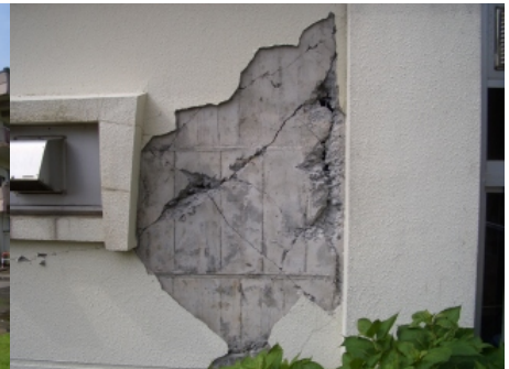
Photograph 27 Shear crack of wall of Shimo-Oguni elementary school (Oguni)
