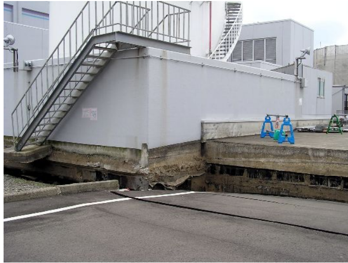
Figure 3 Ground subsidence near the building The building was supported on the bedrock. by courtesy of TEPCO
